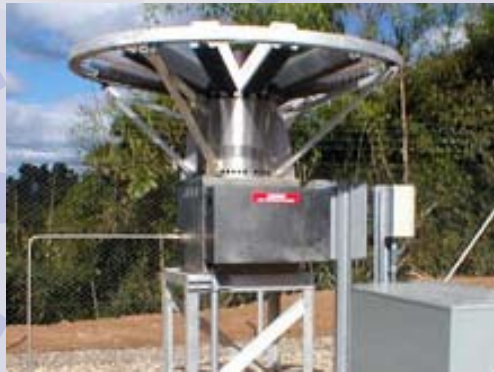
Global TEG on Natural Gas Line, Global Thermoelectric
