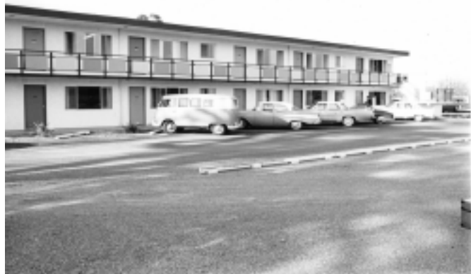
Exterior View, Advanced Systems Development Division (ASDD) Laboratory Annex, Oasis Motel, Monterey Road, San Jose. Two floors and 24 motel units have been converted into offices and laboratories. Photo courtesy of IBM Archives.
