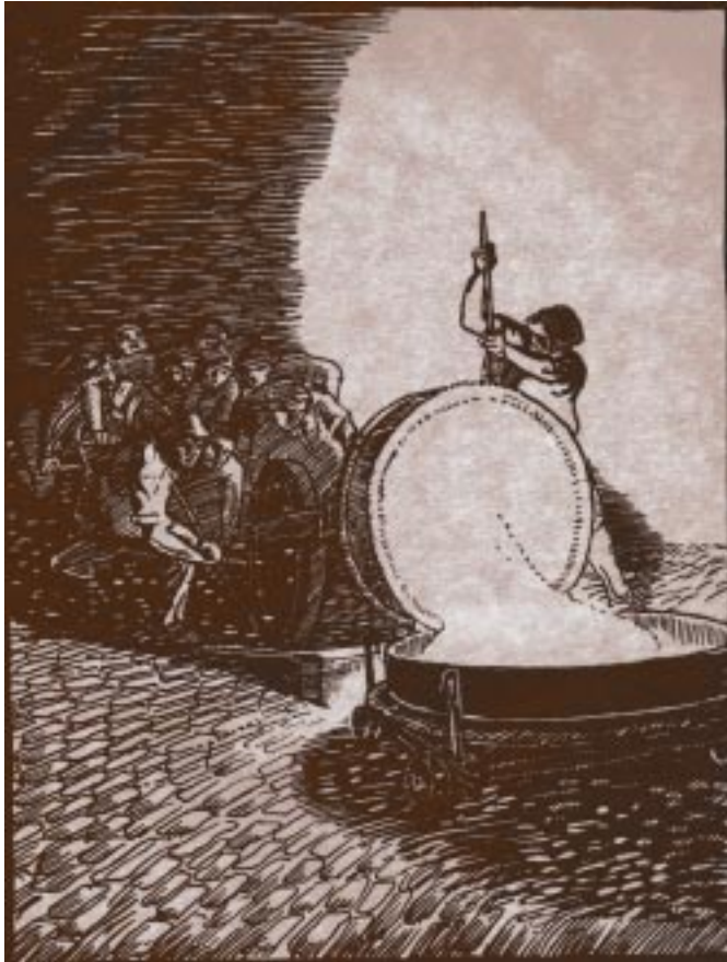
Pouring optical glass in Germany at the turn of the 20 th century, an illustration by Erich Kuithan in Die Glasindustrie in Jena (Jena, 1909). This book turned up during final processing of the papers of spectroscopist W. F. Meggers for the archives of the Niels Bohr Library. The Jena glassworks, created by the physicists Carl Zeiss and Ernst Abbe along with chemist Otto Schott, was a leading supplier of material for spectroscopes, telescopes, and many other instruments.
