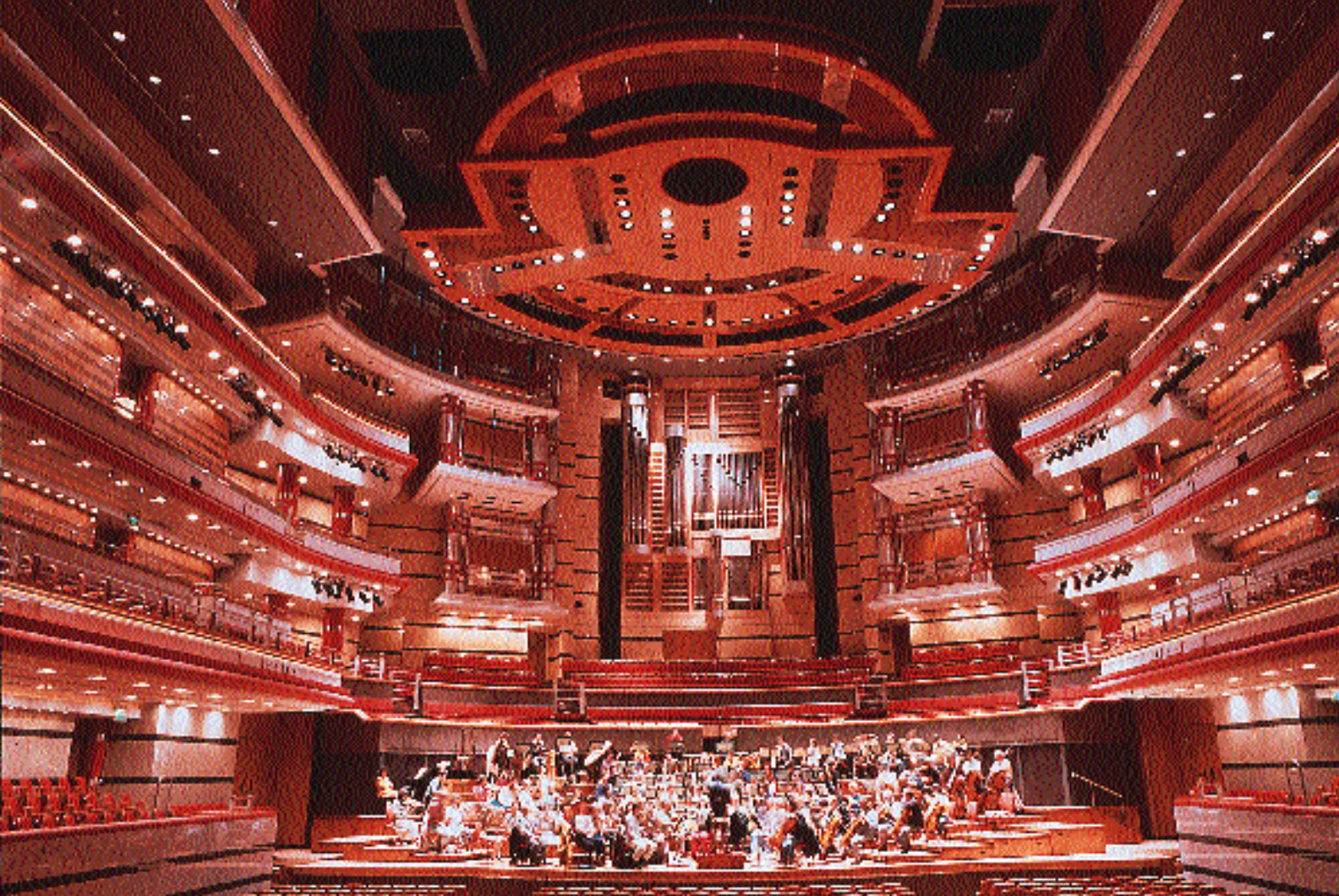
Figure 2. Symphony Hall Birmingham, U.K., which has a reverberation chamber and large adjustable-height canopy, is recognized as having world class acoustics.
